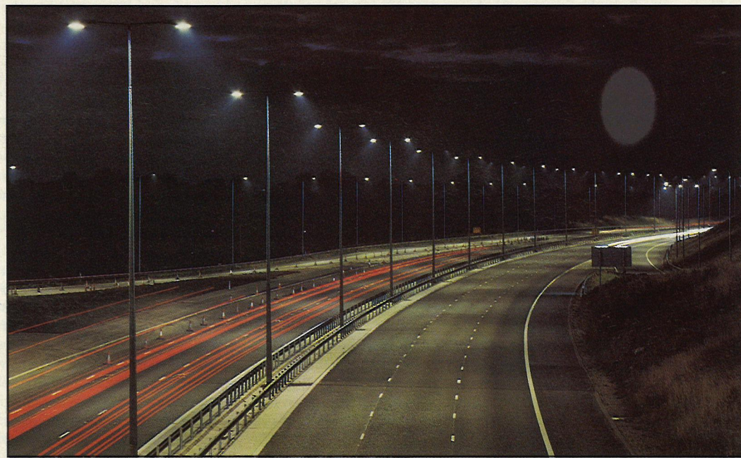
These were replaced by 250W SON/T Plus – which can be changed to 400W if the M5 widens again.
