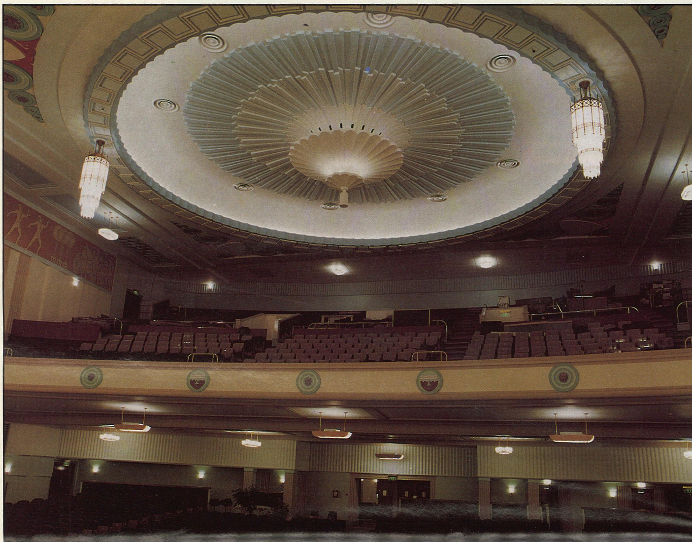
The Bath Forum is a lovingly restored and valuable example of a 1930's grand art deco cinema. The original "Odeon" style luminaires now incorporate a selection of Philips compact fluorescent lamps reducing the installed lighting load by 78% while increasing the illuminance levels.
