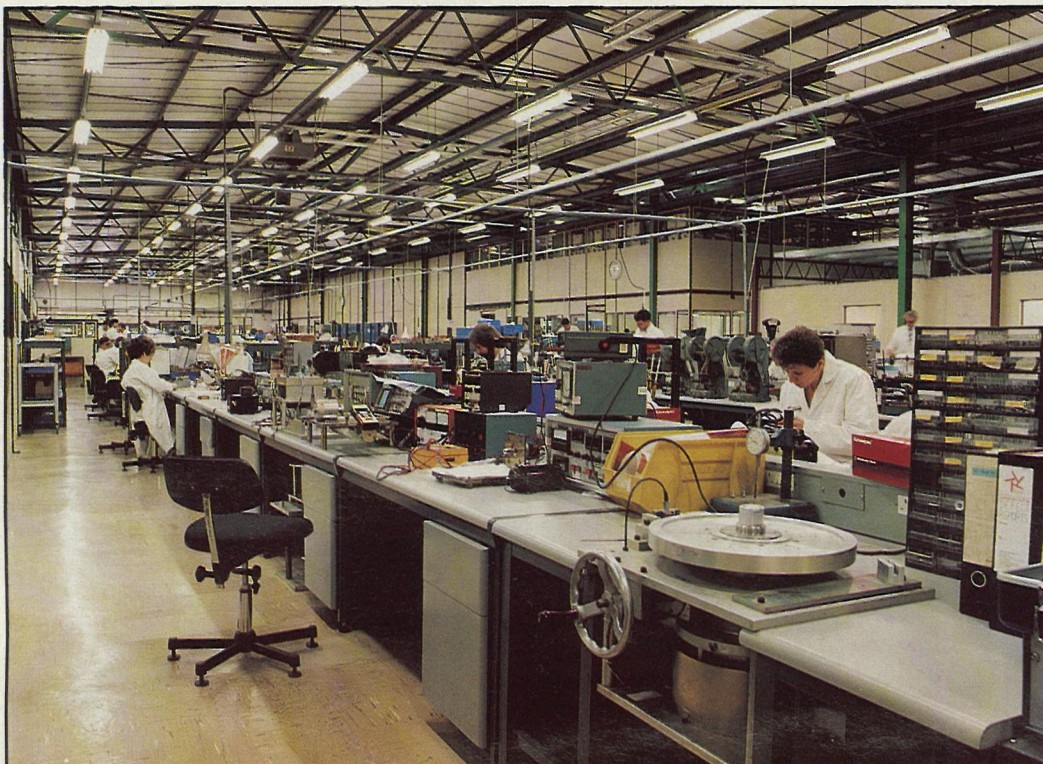
Philips designed the new lighting for Muirhead Vactric Components in Penge using 50W high frequency tubular fluorescent lamps in industrial reflectors. Illuminance levels have been increased by 36% and the power consumption for lighting reduced by 52%.
